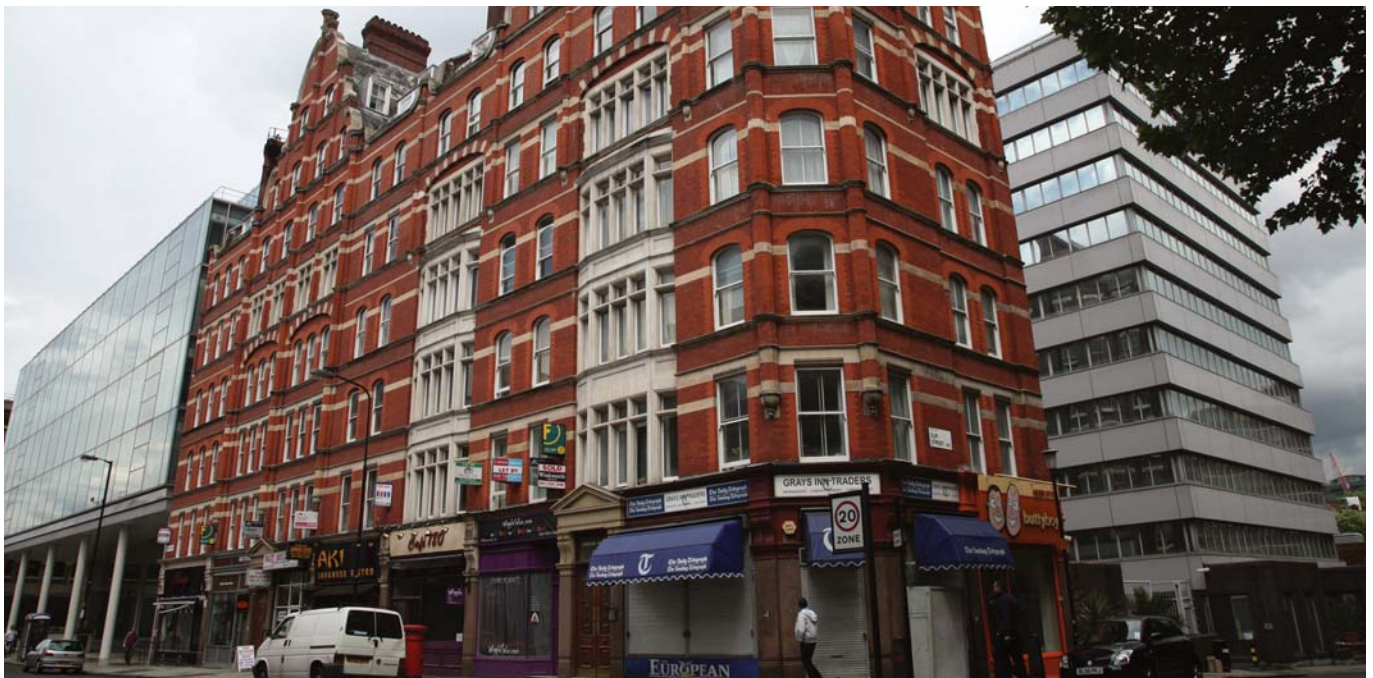
200 Gray's Inn Road (far left) and Elm House (far right)
